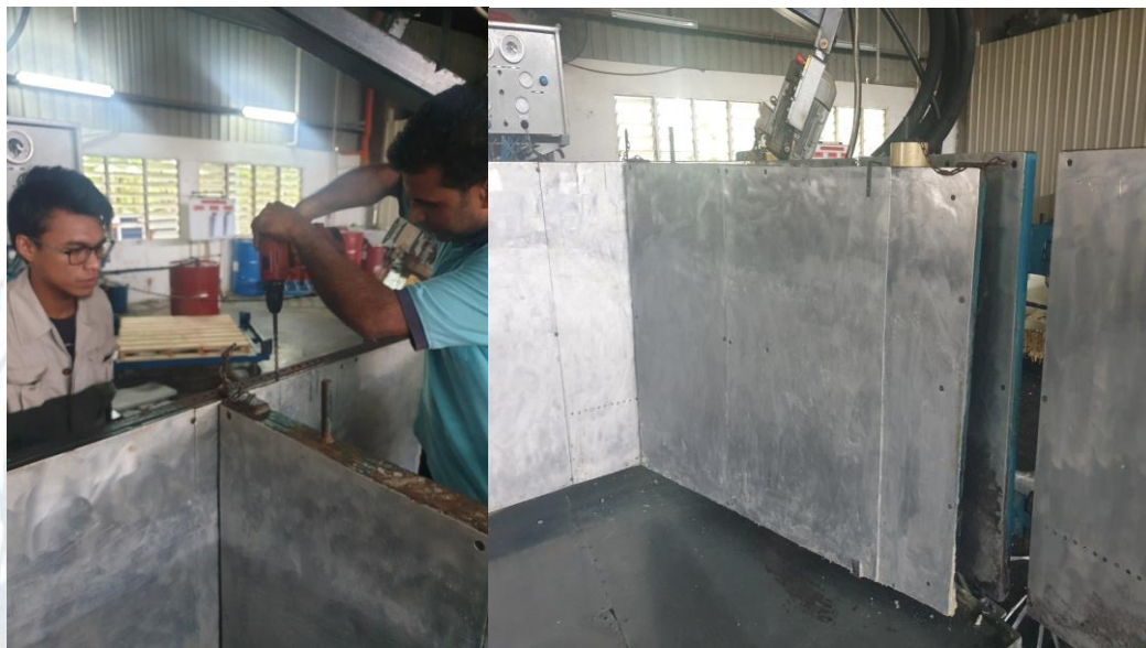
Figure 3 The fabrication and installation of the fixture
